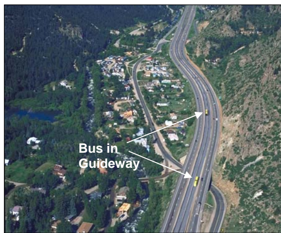
Photo simulation of the Bus in Guideway alternative in the median in Lawson.
